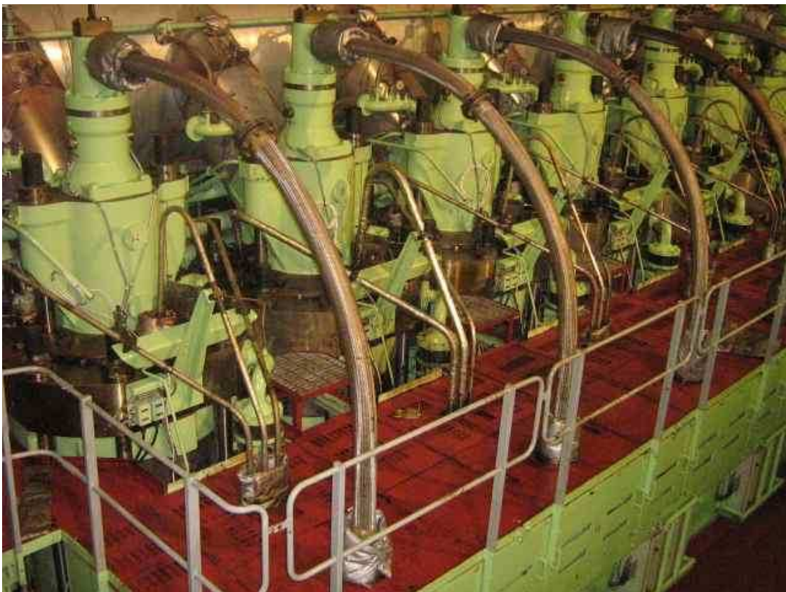
Upper platform of the main engine
